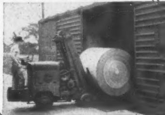
2. The same truck unloads 50" rolls directly from incoming cars and transports them to storage. Rolls are usually stowed in cars two wide and two high.
